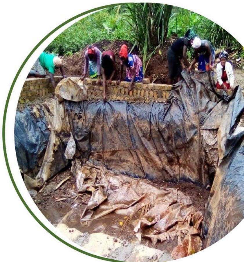
Water pit construction in Uganda. SOURCE: St Jude Family Project
